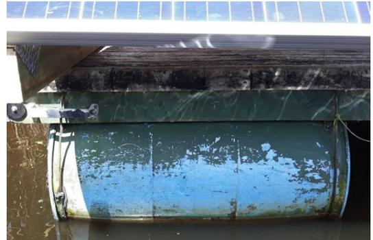
Note our drums had a lip at each end that prevents the stainless wires from sliding off. Locate this drum type if you can.
