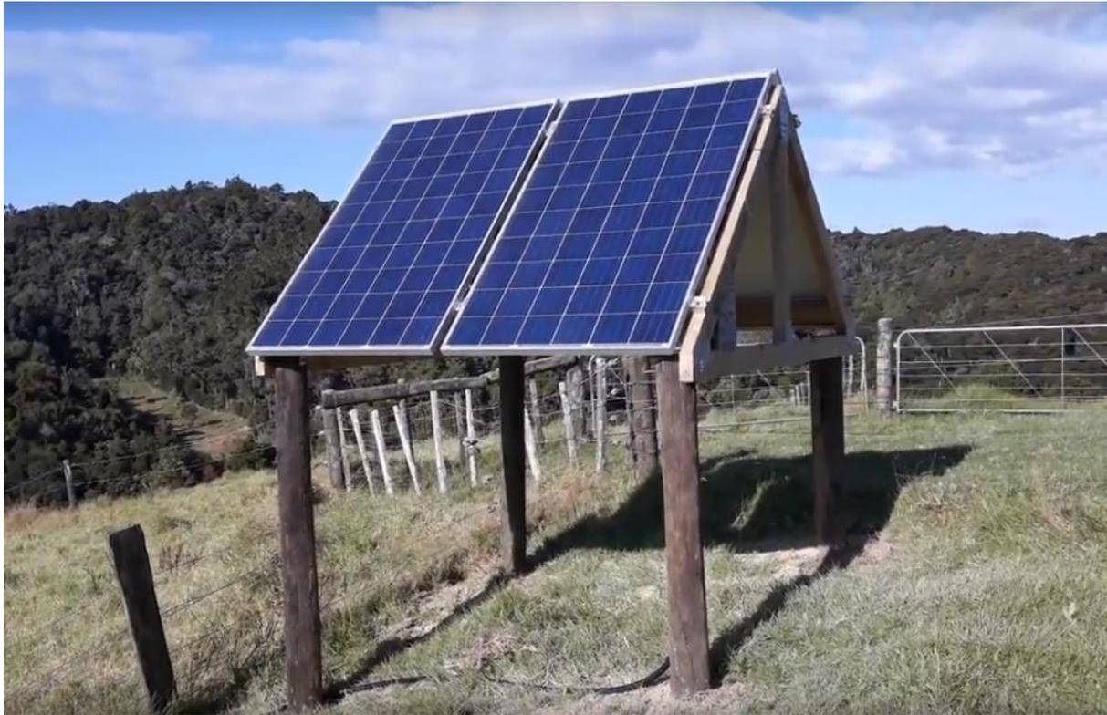
Typical East/West Truss mounted array remote from the RP2 location
