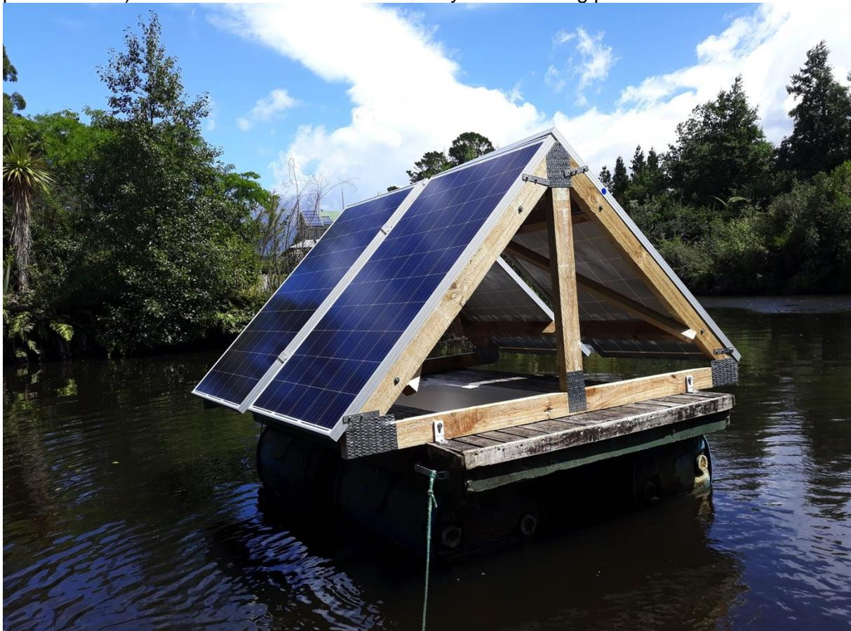
As you can see this works fine, the plastic drums are less than 40% submerged. The trussed frame was then slid onto the pontoon and attached with angle brackets. In this case the panels were attached to the timber frame with stainless steel builders strap. Professional installers are more likely to use aluminium PV mounting rails to replace the timber rails. PV panel mounting is then faster but at higher material cost than illustrated above.
