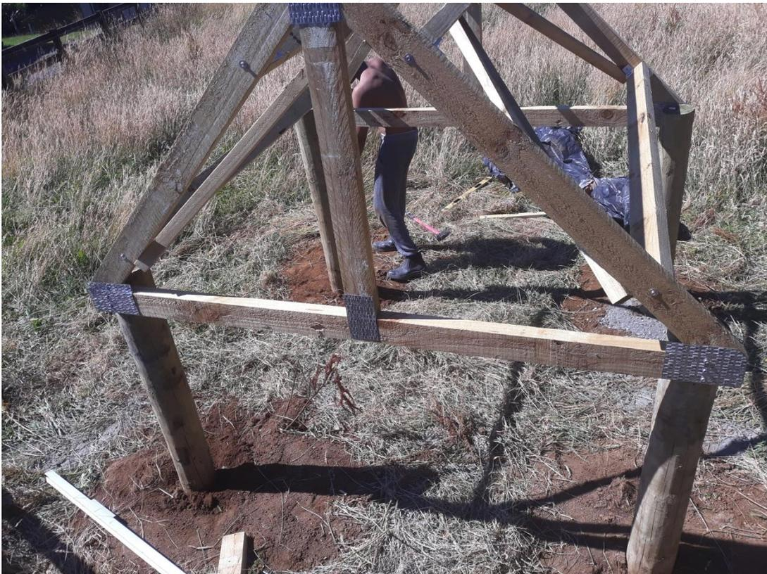
Bolt or use several long Tek screws to secure truss at each post location.
