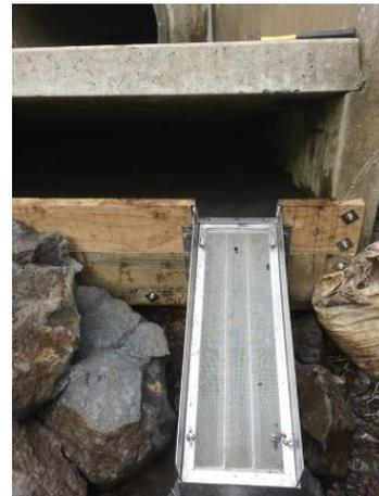
The intake of a gravity feed RP2 should be positioned at the base of a small set of rapids (to allow room for a sloping intake screen as shown opposite). Channel the water flow over the top of the screen, so it falls through the holes into the chamber below that feeds the intake line of the RP2. Leaves and twigs are washed away with surplus water preventing the intake from blocking.
