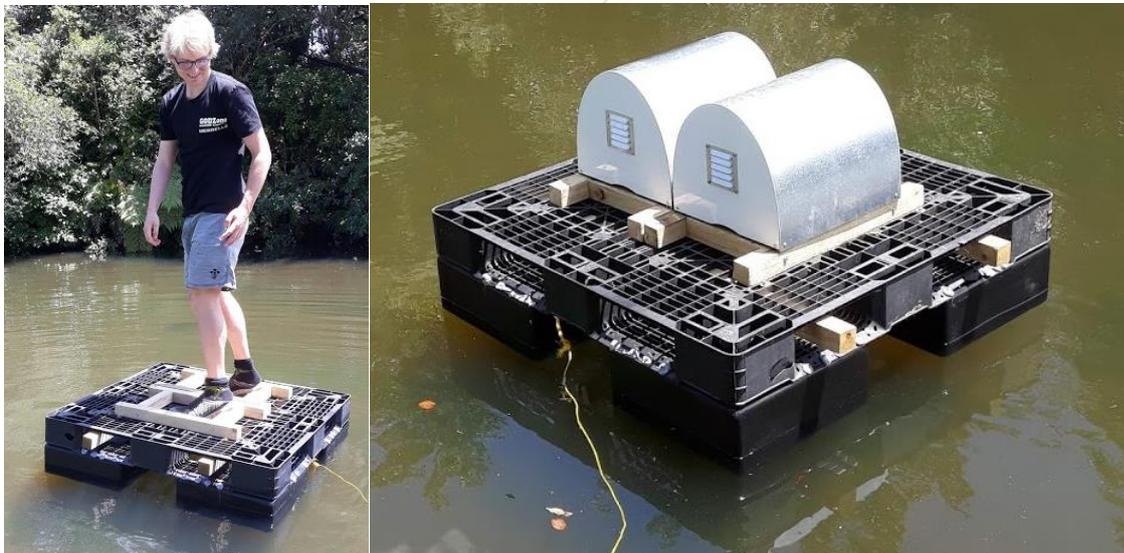
Testing buoyancy of the pontoon prior to connecting: suction pipe, foot valve, filter sock, delivery pipe and power cable
