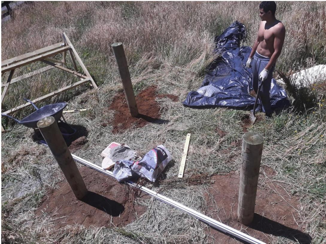
Posts are 2.1m long, 0.9m in the ground and dry mix concrete rammed to secure in place.
