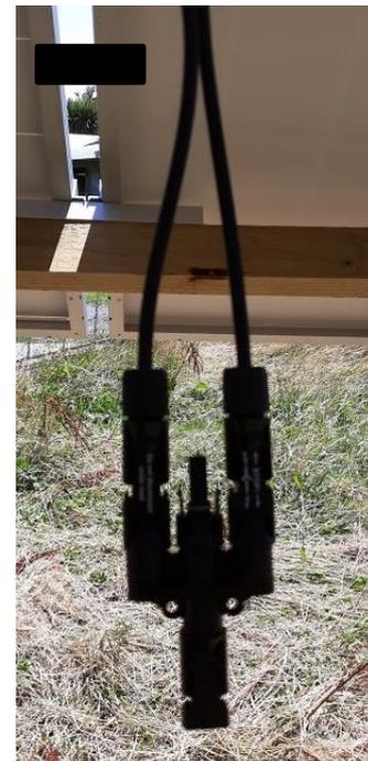
Connect the positive wires into the 2 to 1 Branch connector. Note the connectors shown allows for 3 connections (**6 panel systems are no longer approved as the higher**
