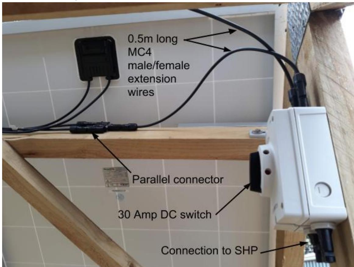
Each RP2 is supplied with a waterproof MC4 DC switch for easy and fast connection as shown above. **Install the DC switch out of direct rain and sunlight.**
